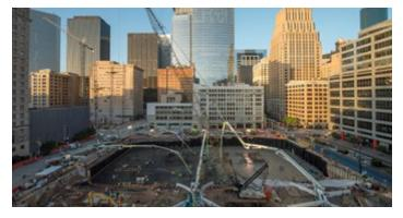
Ceco provided concrete formwork services for this tower and garage project, working with the project team to take maximum advantage of the site's tight downtown footprint. By using wide module pan construction for the office tower, the Ceco team was able to maximize efficiency to follow an aggressive schedule. For instance, Ceco engineers and field forces customized the longform pan system to achieve an eight-day cycle per floor, with each office level measuring approximately 28,000 square feet.
