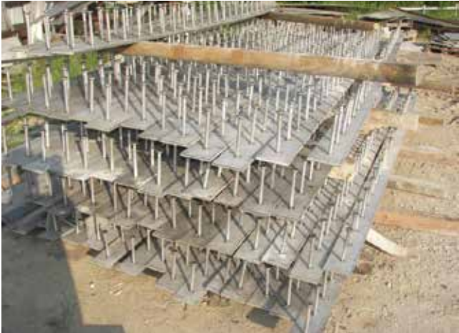
Fig. 8: Embeds must be stored in a designated area and supported on cribbing or pallets. In this example, several of the embed plates are curved, warped, or twisted. Slight imperfections can be corrected during installation once embeds are nailed in place. Note, however, that these plates lack nail holes. If adequate corrections cannot be made, deformed embeds should not be used (photo courtesy of Ceco Concrete Construction)
