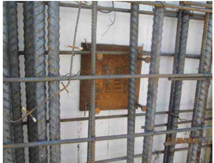
Fig. 6: Embed plates require small diameter holes for installation on wall form (photo courtesy of Ceko Concrete Construction)
